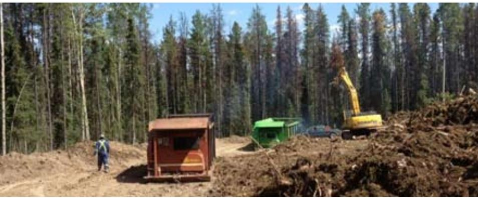
BRE's new air burners are used instead of big burn piles. The new burners greatly reduce air pollution.
